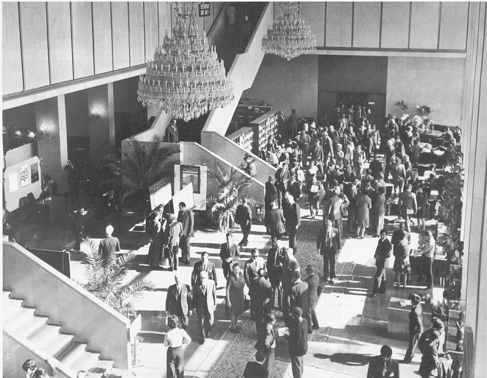
A view of the Majlis entrance hall.
