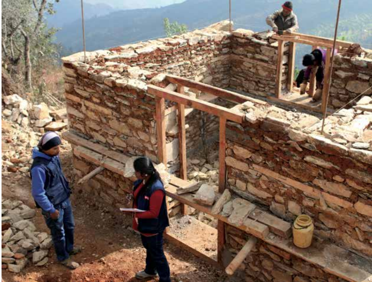
A reconstruction project in Nepal following the 2015 earthquakes that destroyed 91% of the houses in the Ramechhap district. This project seeks to build back better including through masonry trainings and improved building design (Medair).
