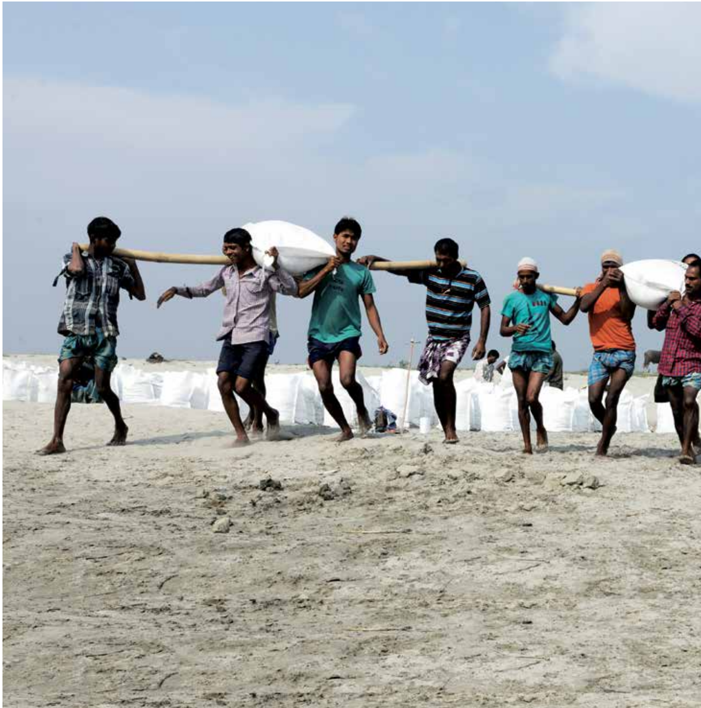
Workers carrying sand bags to be pitched on the banks of the river Brahmaputra in Gumi village, Guwahati, Assam, India. This protects the village from flooding through preventing soil erosion of the riverbank (Asian Development Bank).
