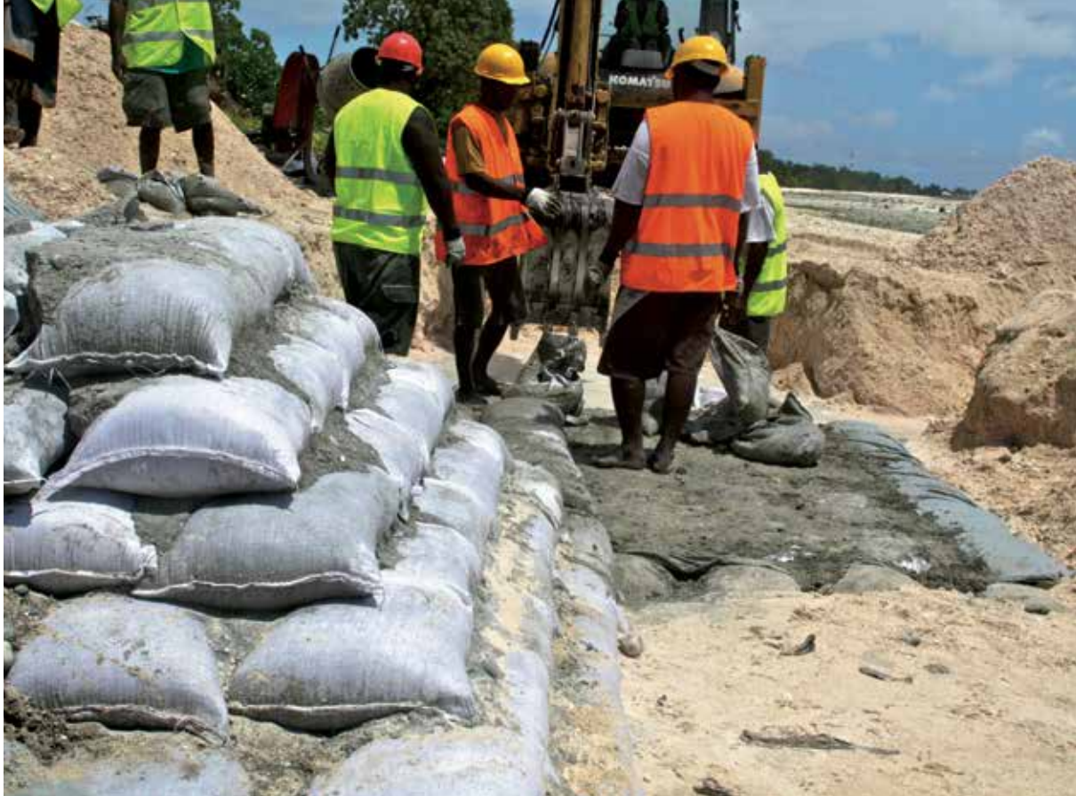
Workers constructing seawalls to prevent soil erosion in Tarawa, Kiribati (World Bank).
